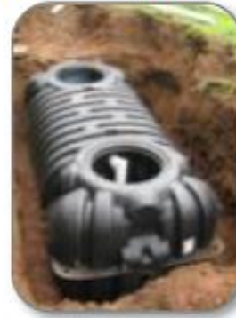
Flush: Septic tank
